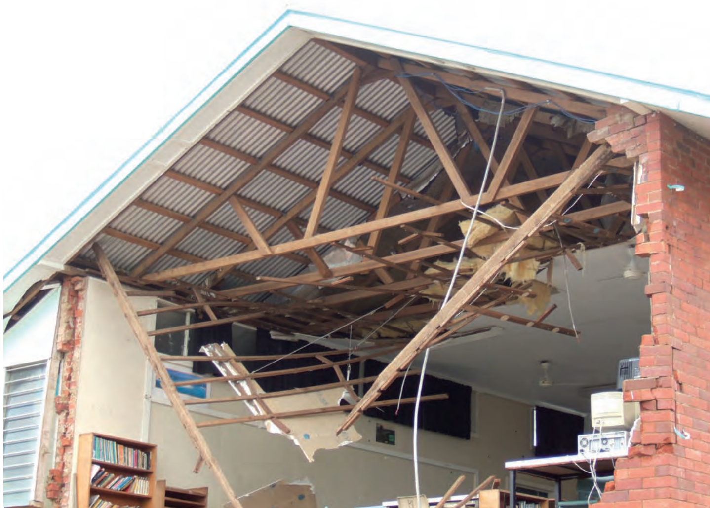
Innisfail State High School built in 1968. Damaged by cyclone Larry - March 2006
