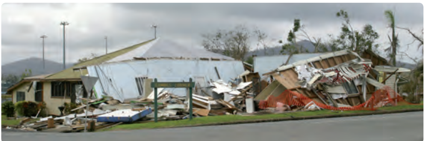
Building damage by cyclone Larry - March 2006
