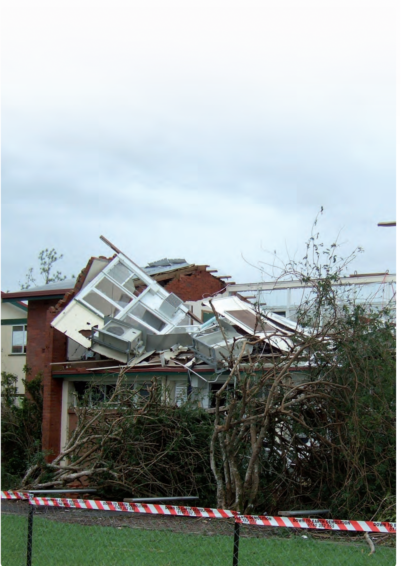
Innisfail State High School built in 1968. Damaged by cyclone Larry - March 2006
