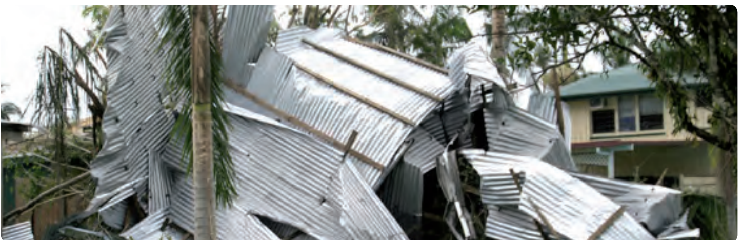
Building damage by cyclone Larry - March 2006
