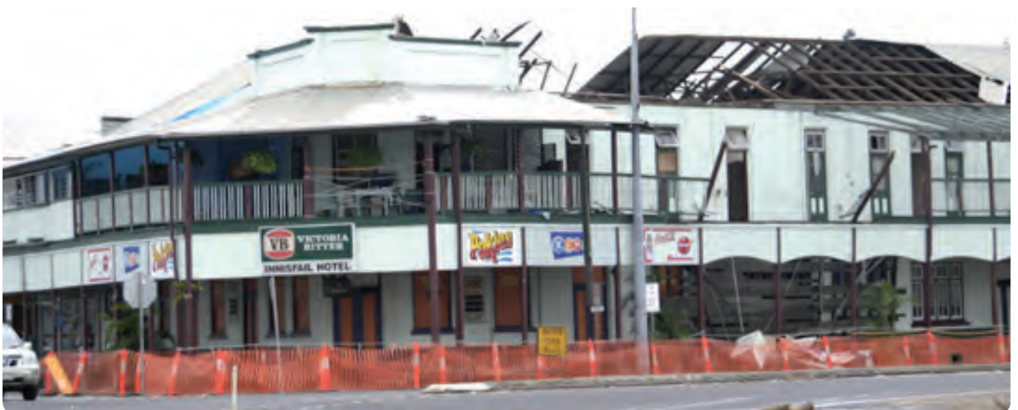
Building damage by cyclone Larry - March 2006
