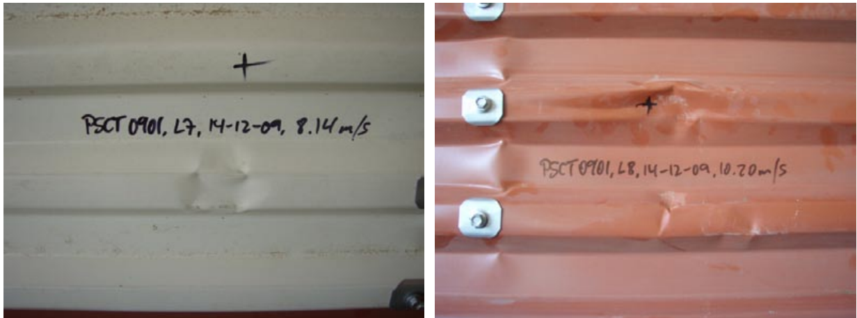
Figure 5: Cladding damage after Trials L7 (left) and L8 (right)
