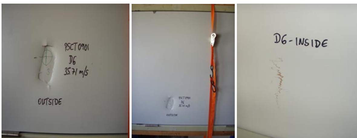
Figure 3: Door damage after Trial SS3
