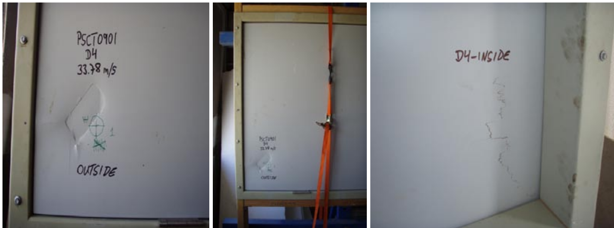
Figure 1: Door damage after Trial SS1
