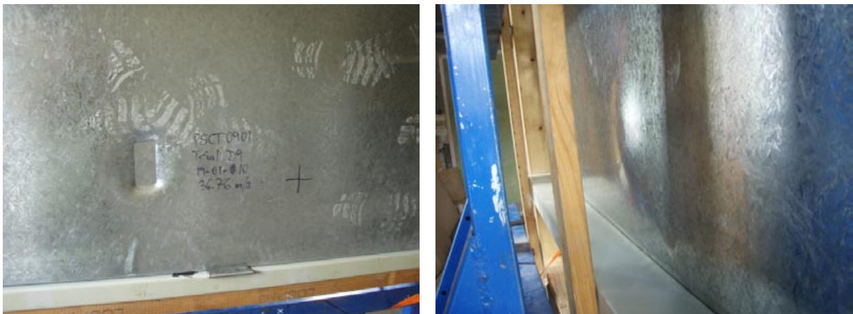
Figure 6: Door damage after Trial SU3
