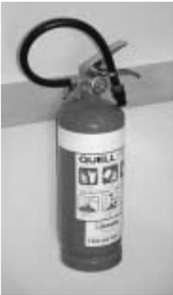
The portable fire extinguishers are to be used by building occupants as a first attack fire-fighting tool on small fires that may occur in the building. They come in several different types to fight different sorts of fires, all of which will require regular maintenance to ensure that they work when needed.
