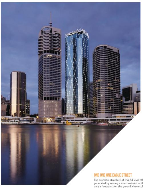
The dramatic structure of this 54 level office tower was generated by solving a site constraint of there being only a few points on the ground where columns could land. The structure reflects two iconic Brisbane fig trees in front of the building, and creates a distinctive identity and spatial experience in the city.
