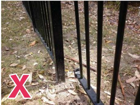
A fence in disrepair can lower the effective height of the barrier or provide a gap for a child to enter the pool area.
