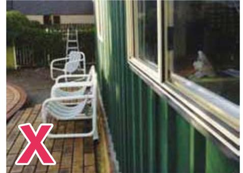
Windows that provide easy access to the pool area must be fixed permanently closed.
