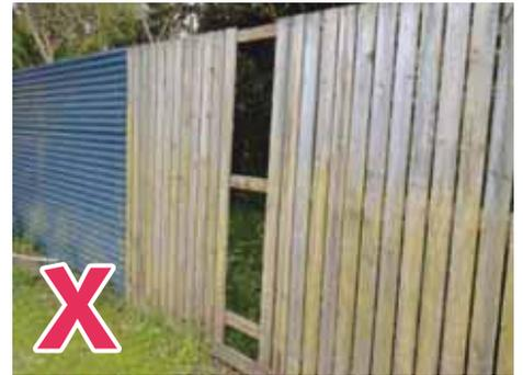
Gaps in a fence over 100 millimetres can provide easy access to the pool area.
