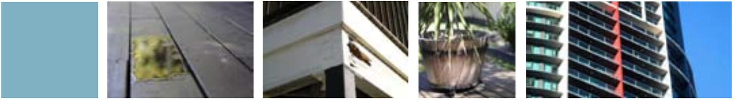
movement from the stress of swaying and twisting under load. Look for warped, cracked or damaged bracing elements and fixings that are loose or deteriorating.
