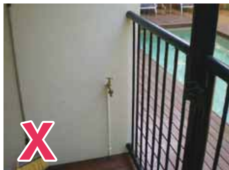
A tap fitting is a climbable object and must be shielded or removed.
