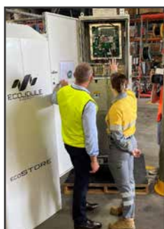
Minister for Energy, Renewables and Hydrogen Mick de Brenni and Energy Queensland Graduate Engineer Emily Shawsmith inspecting two batteries on display.
